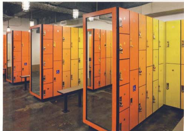
The renovated locker room at the 14 th Street YMHA Jewish Community Center.
